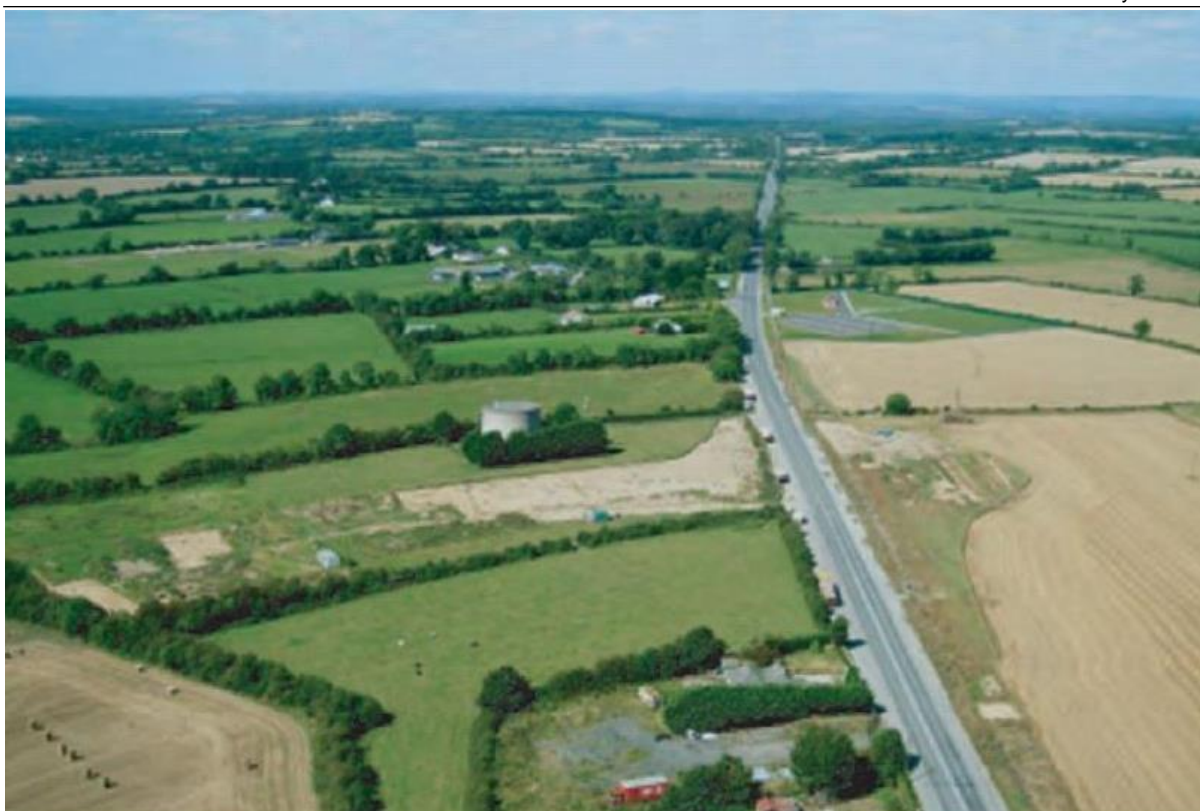
Figure 2-20 - Rath Roundabout and N2 Finglas to Ashbourne Road under construction
